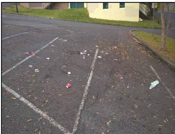
Photograph 9 – Typical representation of the car park surface, cracks/fractures, hydrocarbon staining and litter.
