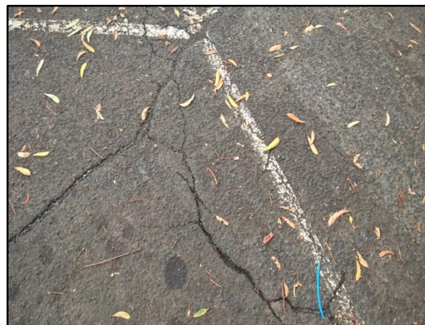
Photograph 10 – Close up of the car park surface fractures and hydrocarbon staining.
